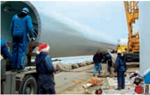
3 The tower bottom section is made ready to be installed.
