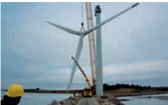
7 The rotor section is mounted to the nacelle.
