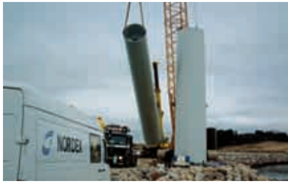
4 The tower top section is being installed.
