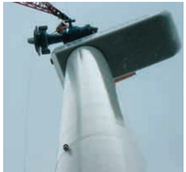
... and thereafter the drivetrain is mounted.
