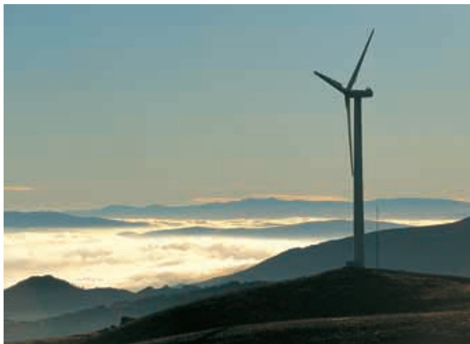
N60 at the wind farm Cabeço Alto, Portugal.
