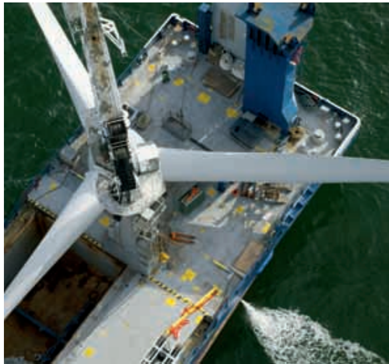
The completed rotor ready for erection.
