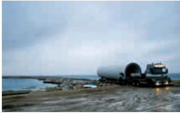
2 It is early morning, and the truck backs on the pier with the tower bottom section.
