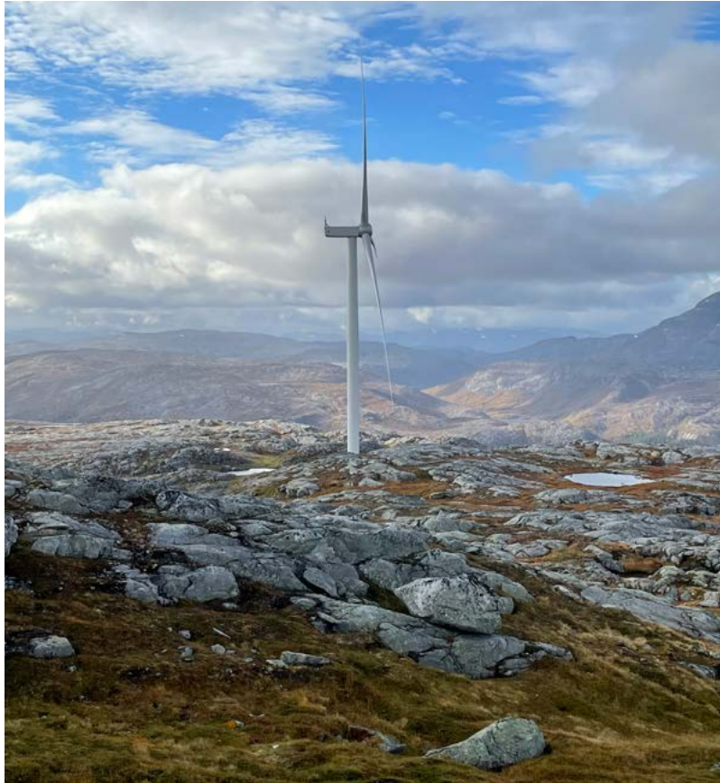
One of 72 turbines, type N149/5.X, for the Øyfjellet wind farm in Norway.
