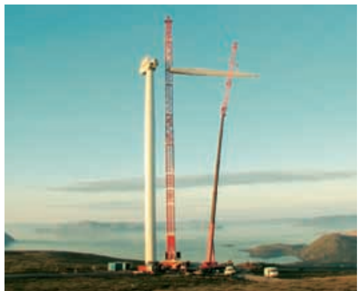
July 15, 2002: The first N80 installed at the site in Norway.
