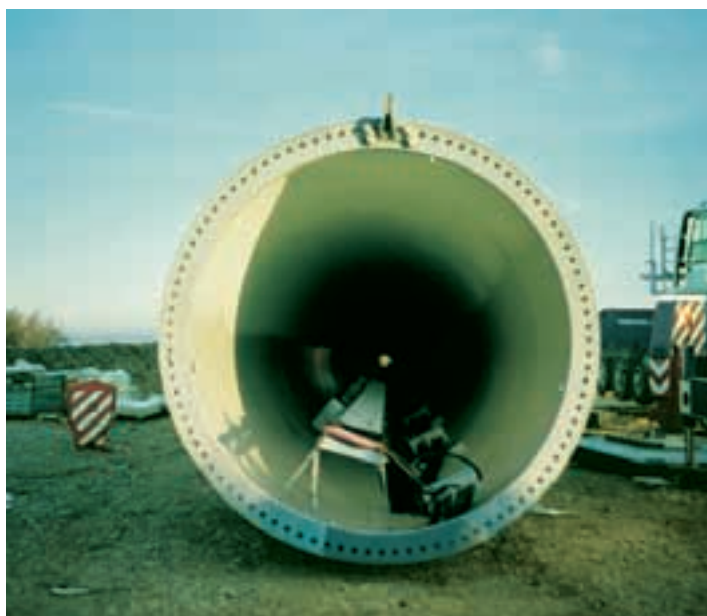
Tower section ready to be mounted
