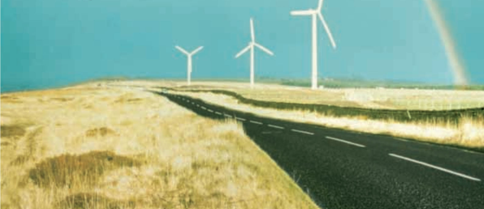
At the end of the rainbow, some of the N50 Nordex wind turbines at the Tow Law and High Hedley Hope projects.
