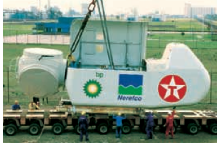
One of the huge N80 nacelles at the Nerefco site.
