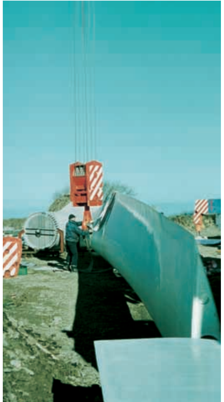
The 29 m long and 5 tons heavy blade prepared to be lifted.
