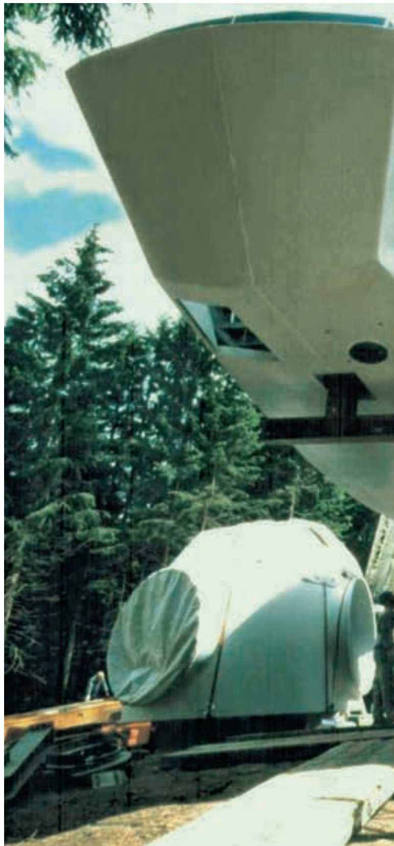
Installation of the S77/1500 kW.
