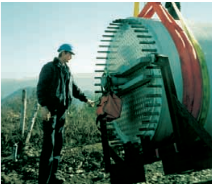
The blade is now ready to be mounted to the hub
