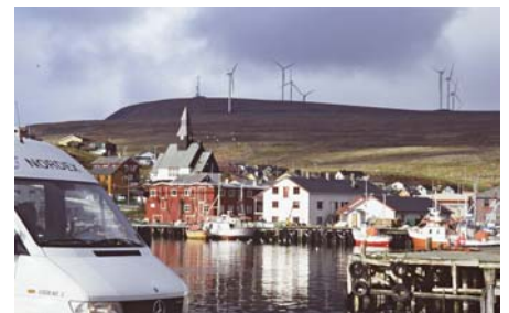
The N80s erected on the beautiful site in Havøygavlen.
