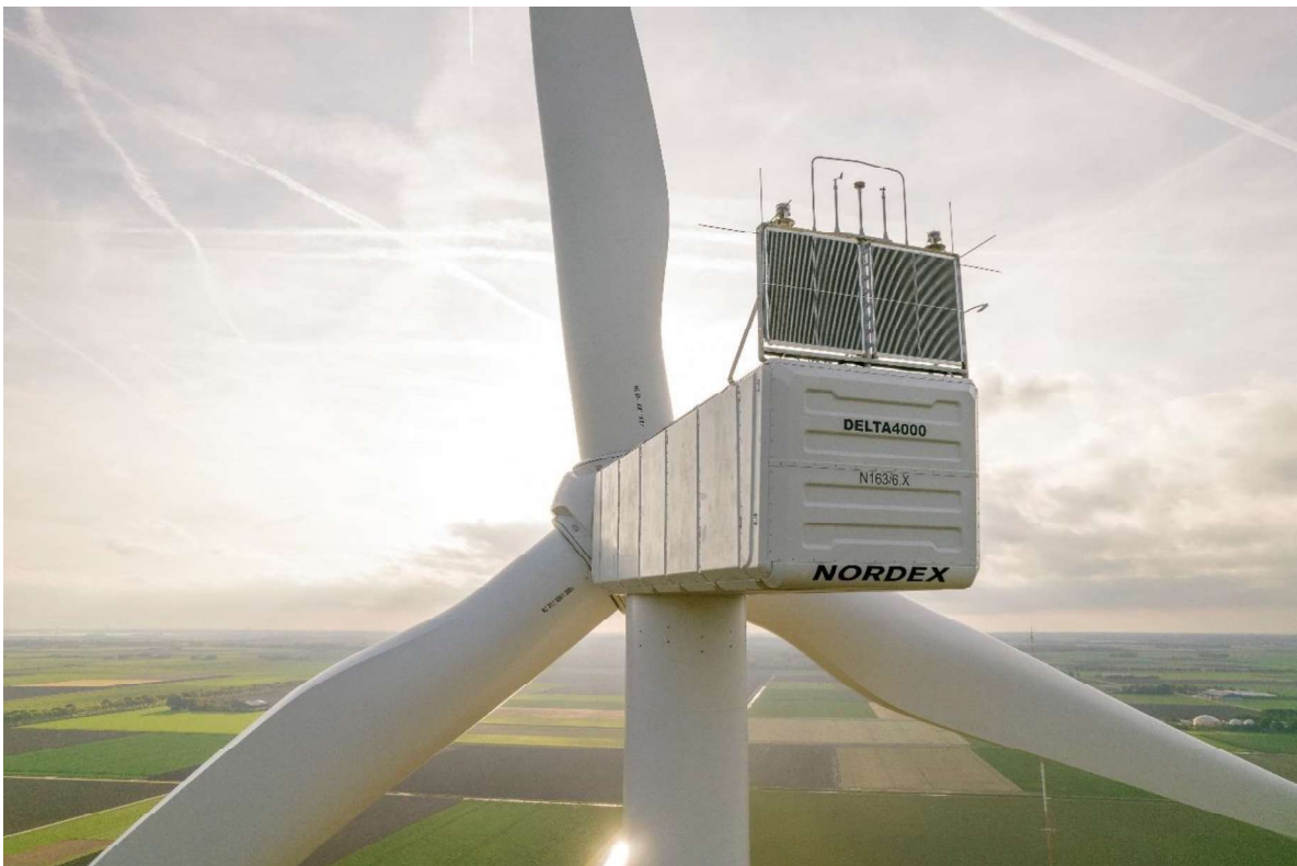
Figure 1: Product system – view of Delta4000 N163/6.X turbine
