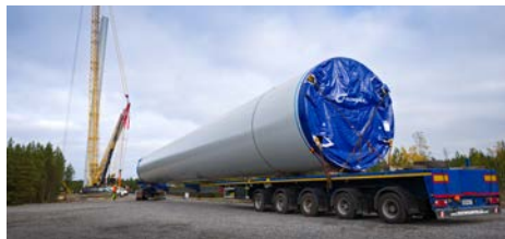
Low-emission steel is one of the most impactful measures for reducing greenhouse gas emissions in Nordex turbines. The image shows an exemplary installation of a Nordex steel tower.
