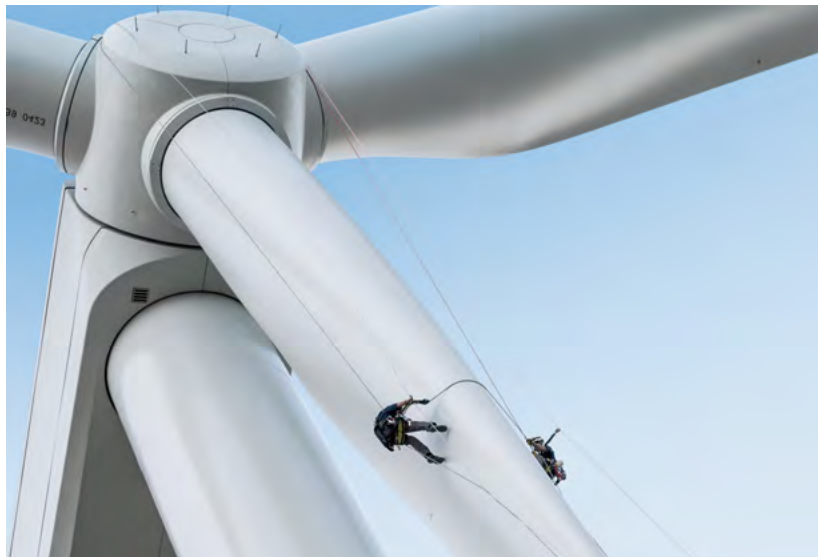
Safety First! Service technicians inspecting rotor blades.
