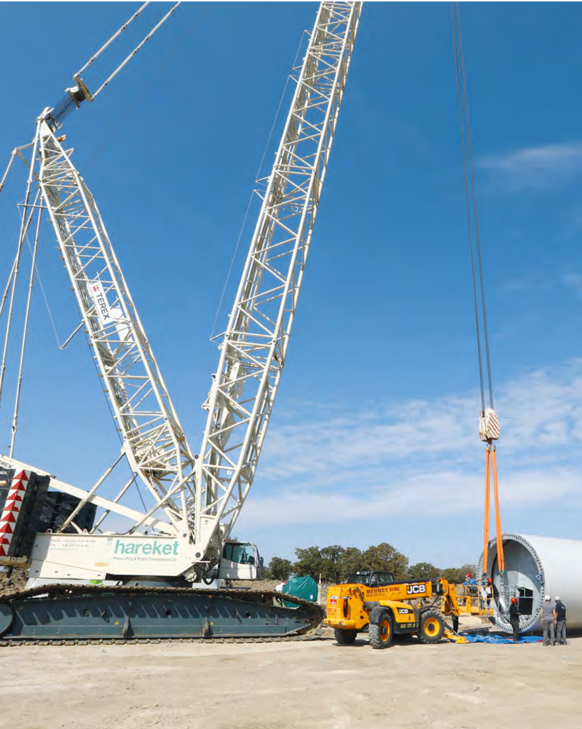
Construction of a Nordex wind turbine in Turkey.
