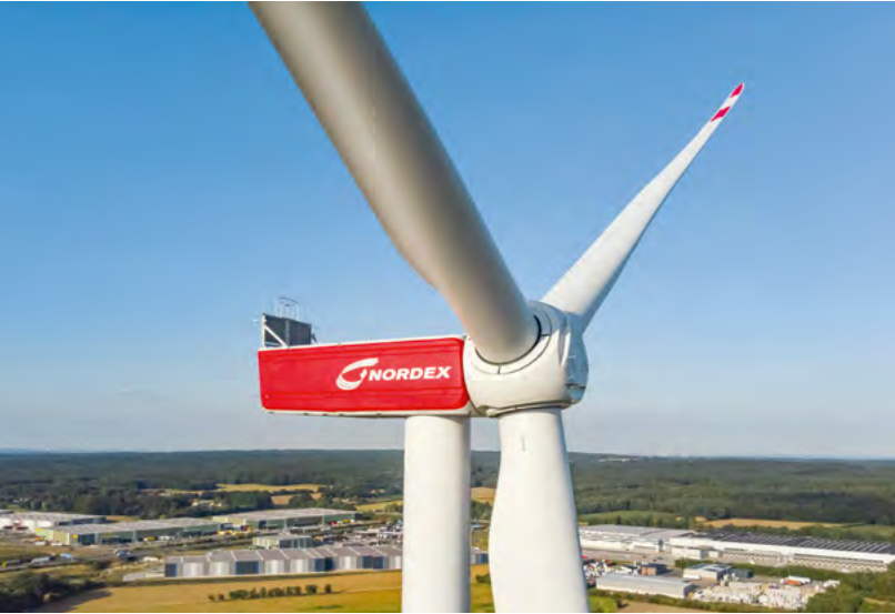
Nordex Delta4000 N149/4.0-4.5 wind turbine in Germany.
